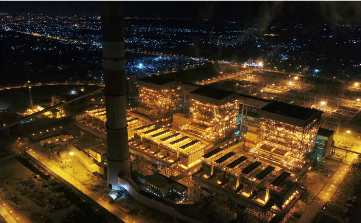
Koradi Thermal Power Station
