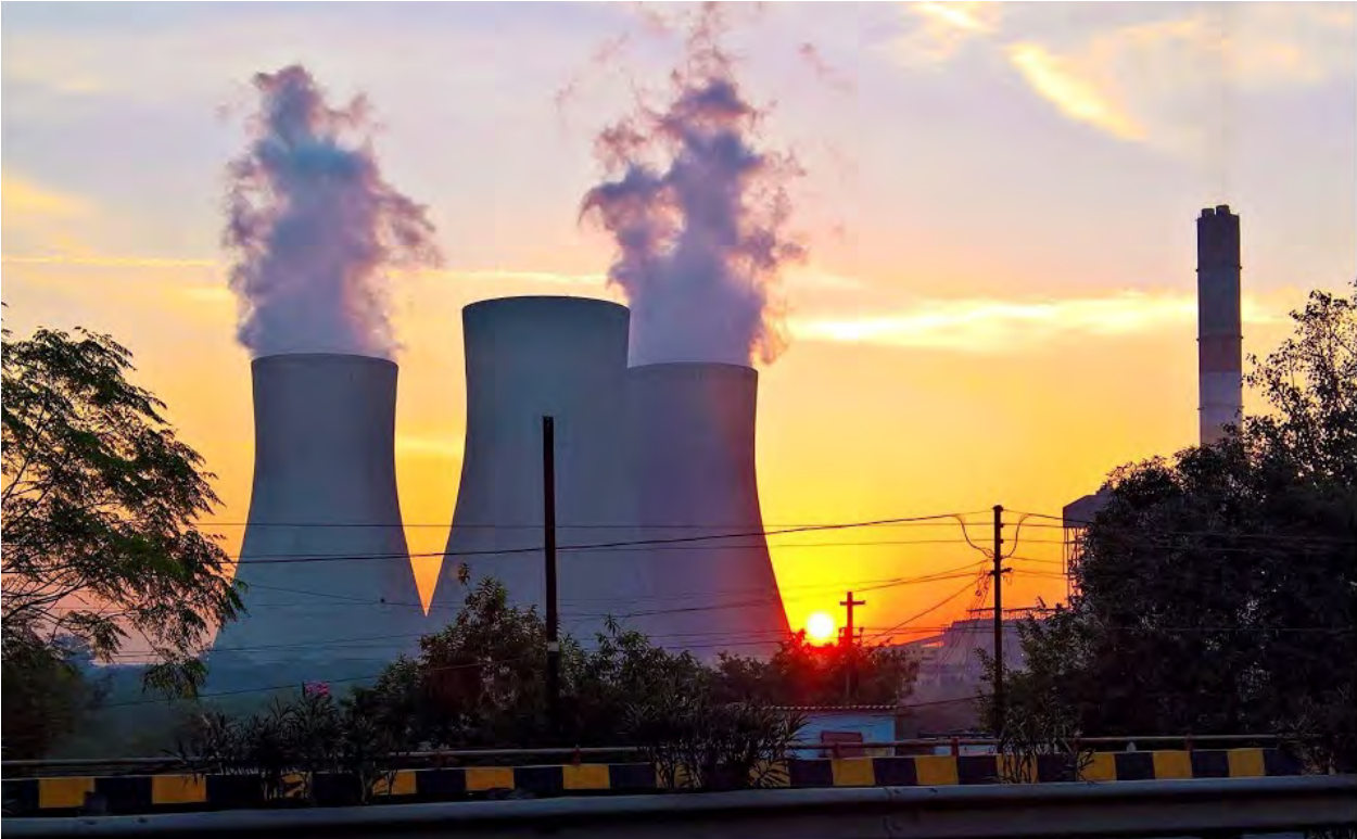
Koradi Thermal Power Station
