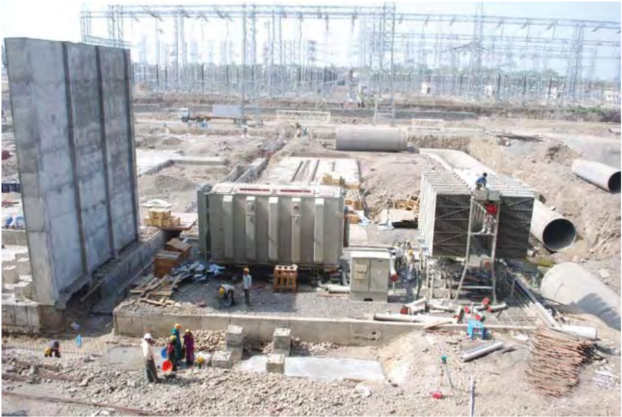
Transformer Foundation Unit No. 4 (Bhusawal Project)
