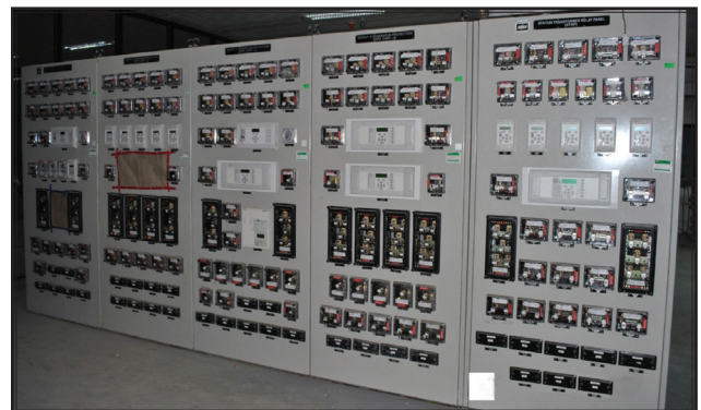
Bhusawal Station & Gen. Transformer Protection Panel Unit 5 (2x500 MW BSL Project)
