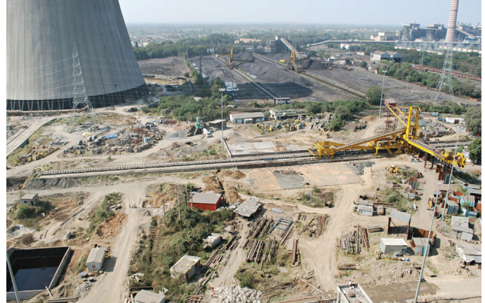
Khaperkheda Stacker Reclaimer (1x500 MW Unit No 5)
