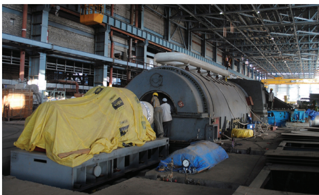
Bhusawal Motor & Stator Unit 4 (2x500 MW BSL Project)
