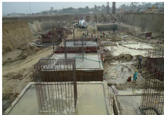
Koradi Turbine Foundation Unit No. 9 (3x660 MW Project)
