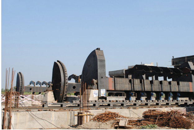
Bhusawal Wagon Tippler 1,2&3 CHP (2x500 MW Project)
